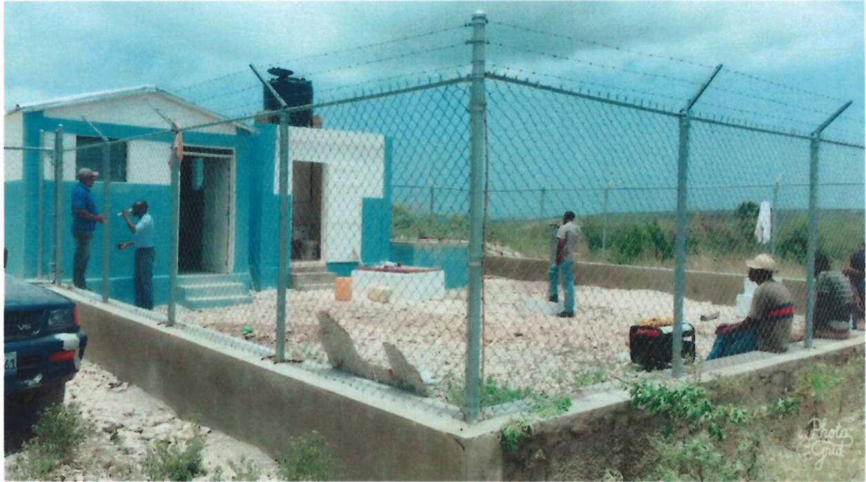
Seismology station in Môle St-Nicolas, North-west
